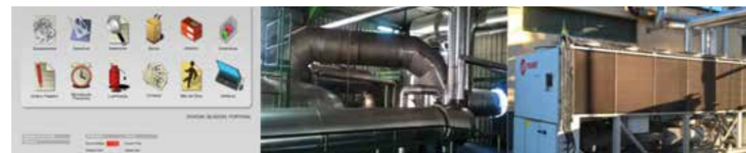
SW Maintenance Management System (Almada)
